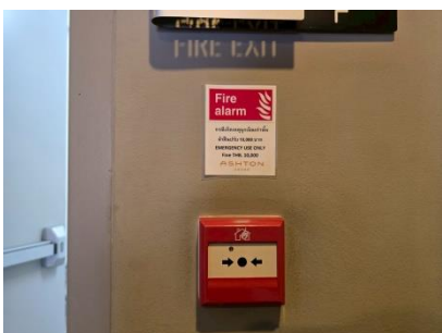
Fire Alarm Manual Station
