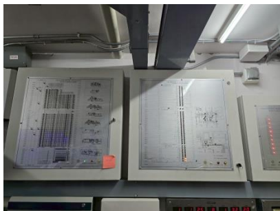
Graphic Annunciator Fire Alarm
